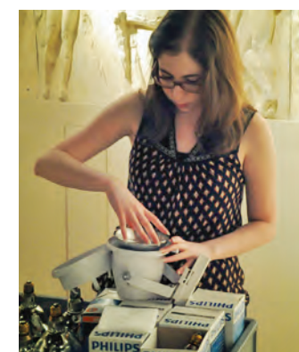
Student employee, Scarlett Andes, installs LED bulbs in light fixtures to be installed in gallery track lights. A total of 1,140 gallery lights were upgraded during this process, both inside cases and in room-ambient light fixtures.
