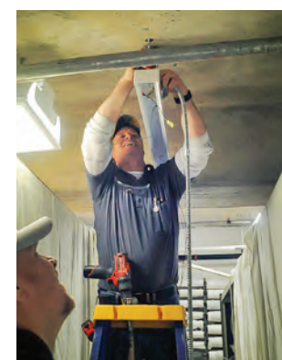
Electricians, Brad Eveland and Doug Dahl, prepare conduit to install an LED light fixture in the Artifact Preservation Center. Sixty-three florescent fixtures were upgraded to LED during this process.
